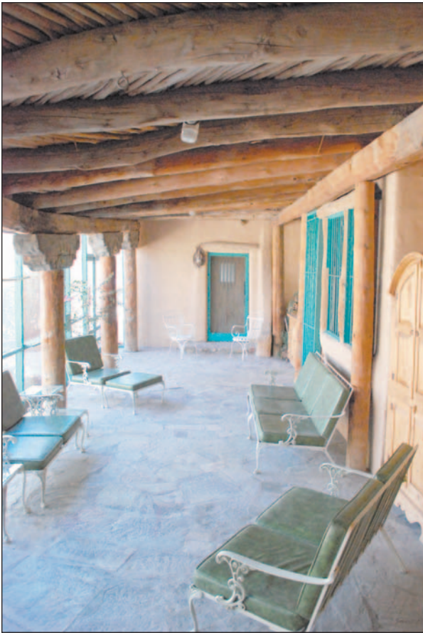
Built in 1887 and purchased in 1902 by Judge Numa and Clara Frenger, the home at 331 W. Las Cruces Ave. was changed to feature a pueblo revival style, which can be seen in the enclosed patio that includes vigas, columns and lintels.
