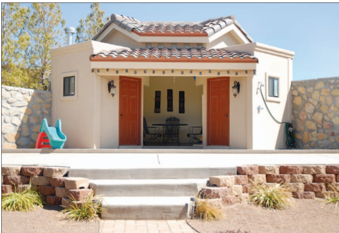
A pool house accompanies the sports pool, which is three-and-a-half feet deep.
