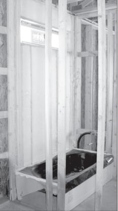
When determining the thermal bypass, or tightness, of a home's envelope, the insulation of the framing and how well it is sealed is examined. This process is part of the El Paso Electric Energy Star New Home Program.
