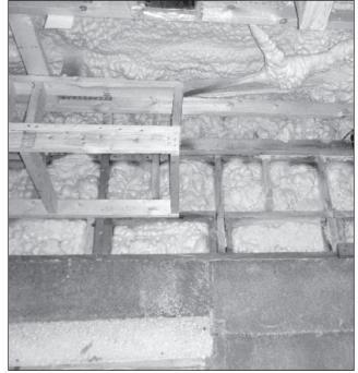
The interior of this roof deck in a Coyle Builders home in Mesilla Hills uses open cell spray foam insulation installed by New Era Air Tight Spray Foam.
