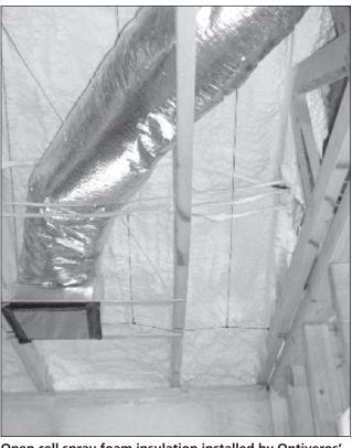
Open cell spray foam insulation installed by Ontiveros' Insulation was used in the non-vented attic space of a Schueller Homes product to seal the home's envelope.
