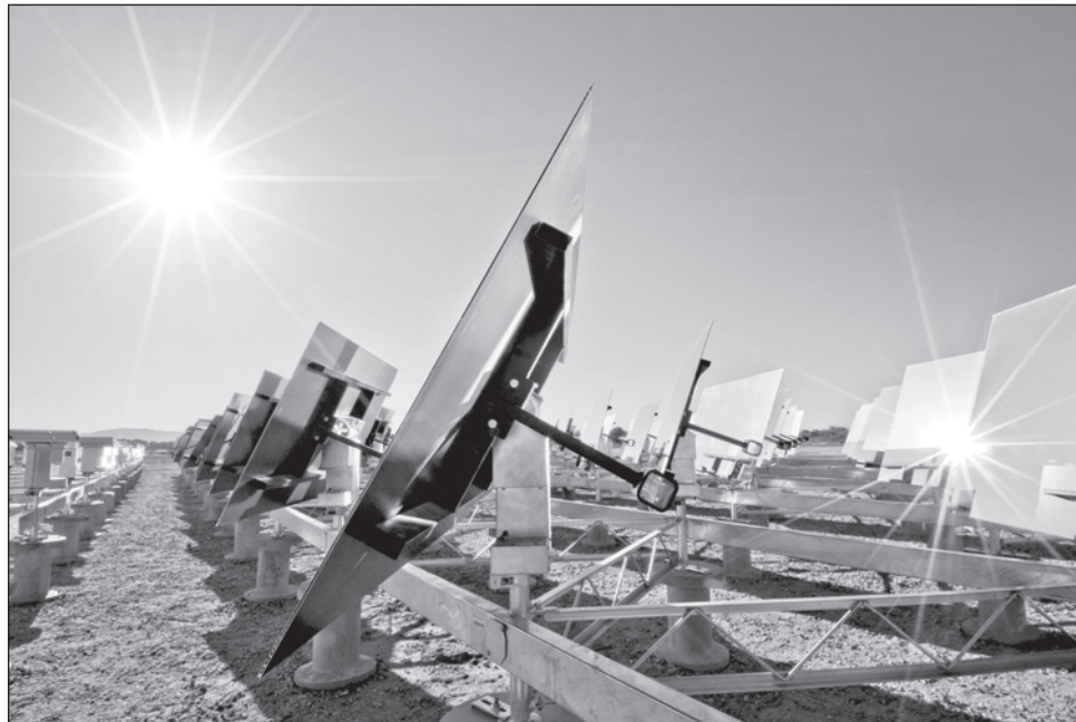
A field of eSolar sun-tracking heliostats absorb energy from the sun. The eSolar heliostats, which concentrate sunlight into a thermal receiver mounted on solar power towers about 180 feet high, will be part of eSolar's facility in Santa Teresa, N.M., as part of power generation partnership with El Paso Electric Co. reached in 2010.
