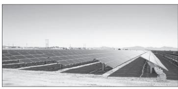
Rather than using solar-thermal technology as originally planned, the NRG Energy Inc. powergeneration facility will use traditional photovoltaic cells such as these in its Blythe field facility in southeastern California.
