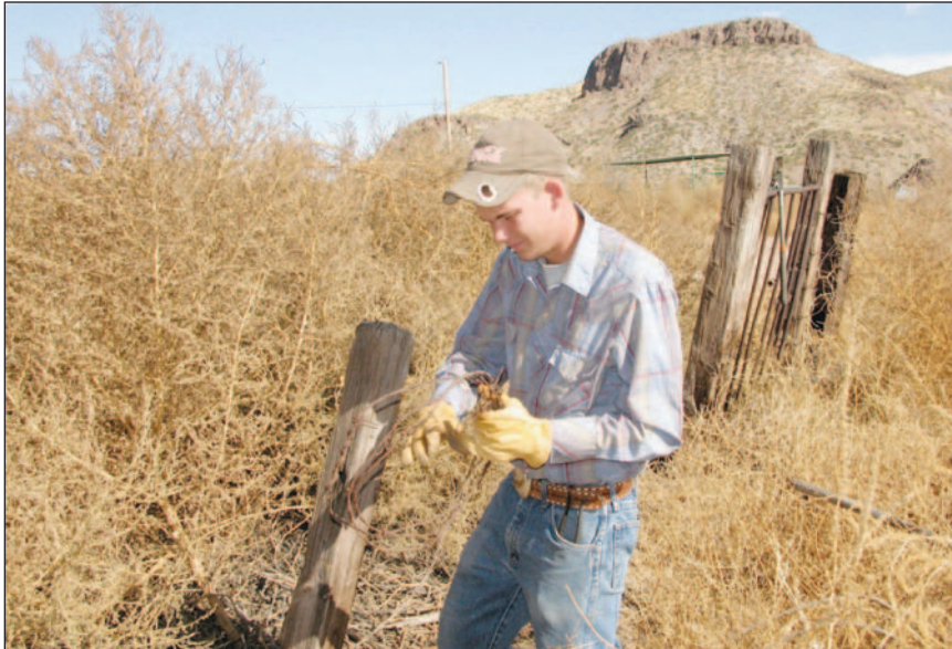
Grant Keever, 17, helps remove the last strand of barbed wire from a fence line Saturday, Nov. 20, for a habitat restoration project at Broad Canyon Ranch, which is part of the New Mexico State Parks system.
