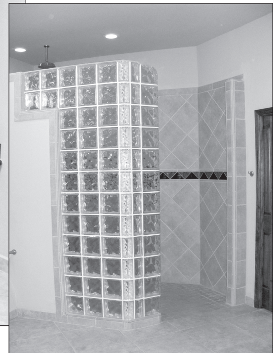
Below: The Straetzes also put in a shower large enough for Susan's wheelchair.
