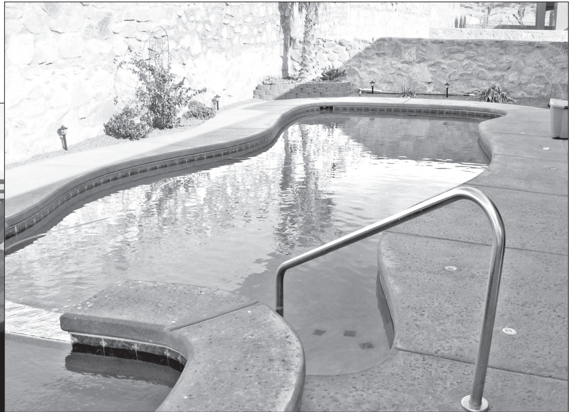
The pool was also made accessible to Susan Straetz, with anchors for a built-in ramp to help her get into the pool.
