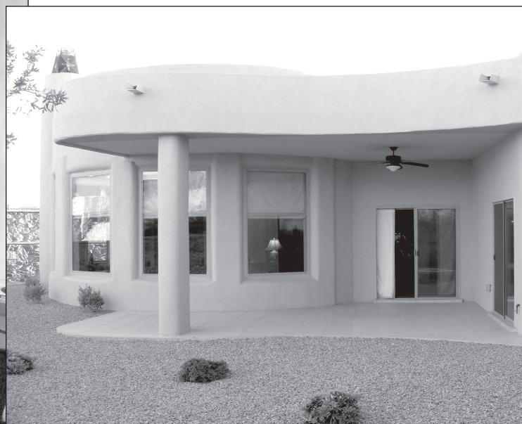
From the backyard one can see the cylindrical living room.
