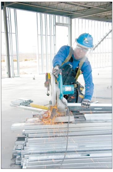
Sparks fly as framer Joe Acosta cuts galvanized steel to make box headers for windows in the new branch of First Light Federal Credit Union at 3791 E. Lohman Ave. The branch is scheduled to open in early Mav.
