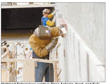
Highland Enterprises welders Tizoc Antonio, front, and Kyle Obyrne weld ledge angles to metal plates in the concrete walls of the Roadrunner Storage facility now under construction at 170 Roadrunner Parkway. The ledge angles will give support to the second floor of the building, when it is put in place.
