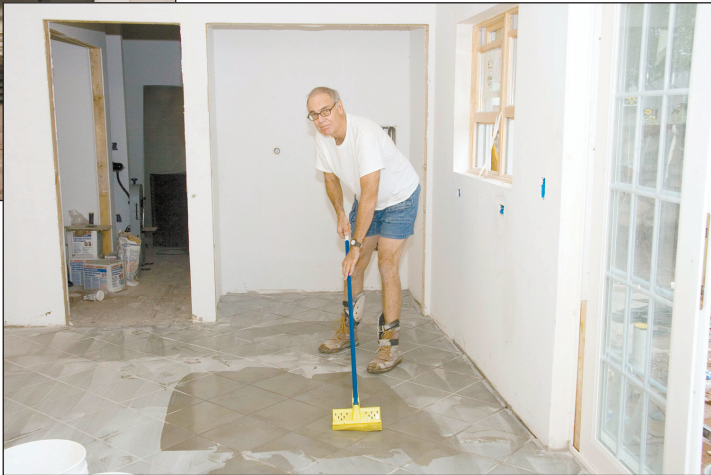
Ron Billingsley cleans up the grout from the new tile that was laid down in the kitchen.
