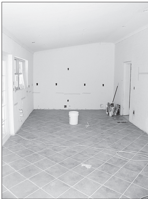
With non-original walls knocked down, the kitchen emerges as a large, sunny room. The partners put in new tile floors.
