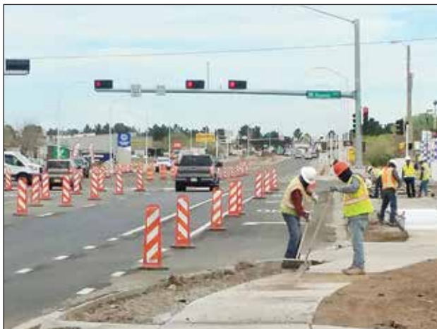
Crews finished the sidewalks and landscaping in May.
