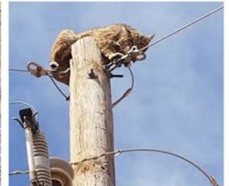
Bobcat on EPE electric pole along Topaz Road.
