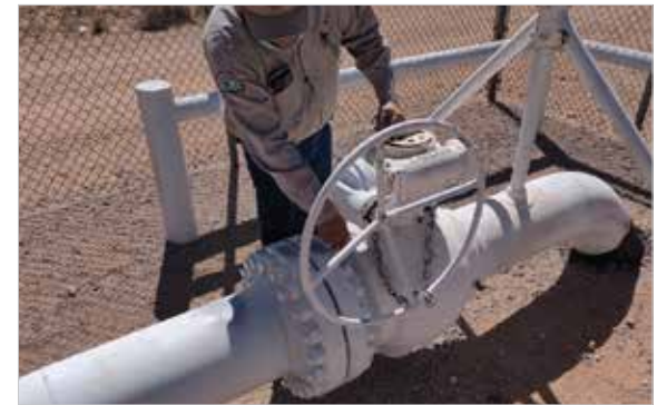
LCU Associate working high-pressure natural gas line—Courtesy LCU
