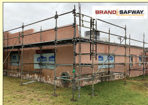
Brand Safway of El Paso, Scaffolding
