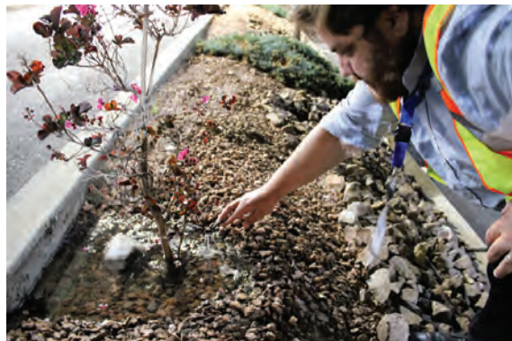
LCU Customer Service Representative William Wilkinson finds a broken irrigation component for a commercial complex at night. LCU will be doing audits to watch for water waste, even during the winter and at night.
