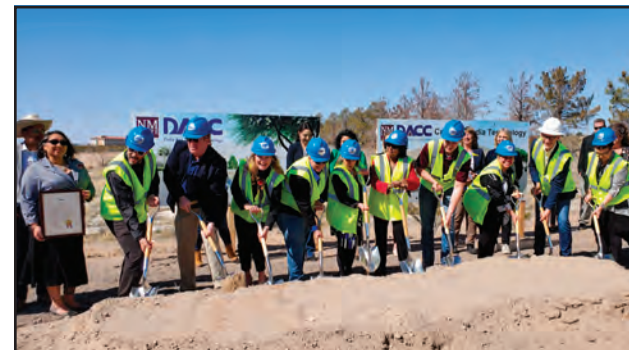
On the site of this groundbreaking, in a little more than a year, will be a 14,000 square-foot building with classrooms and a soundstage, the first phase of the Las Cruces Creative Campus.
