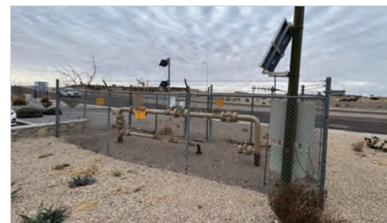
LCU corrosion survey equipment at a test location - Courtesy LCU
