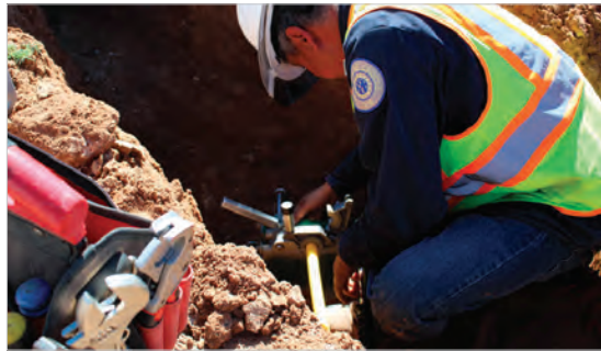
PHOTO 1: LCU team member working on a natural gas line - Courtesy LCU
