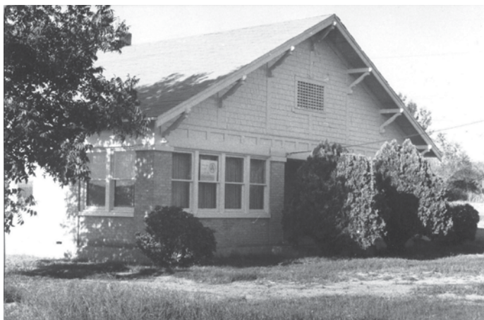
First Branch Main Office Doña Ana County Occupational Education Branch on the corner of University and Espina
