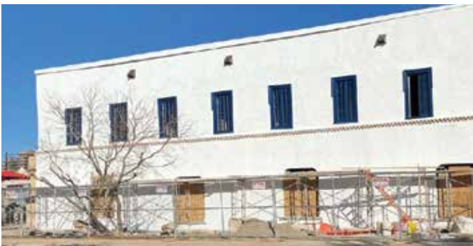
Restored west wall of the Amador Hotel.
