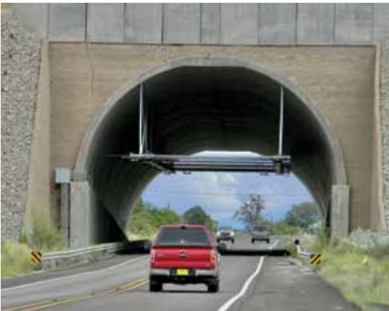
Roadway spans state highway, giving loaded dump trucks access to other sites in the Chino mining complex.
