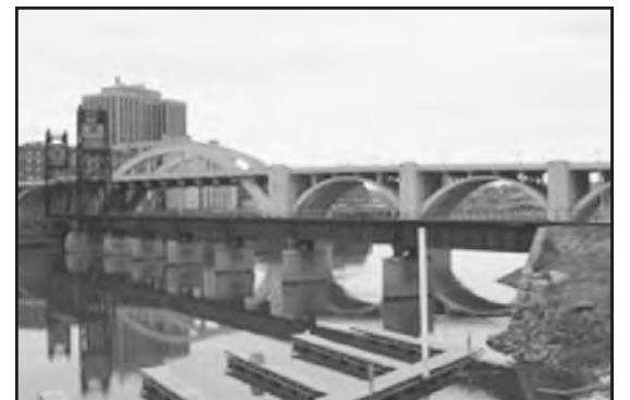
The Robert Street Bridge, St. Paul, designed by Toltz, King, and Day and also on the National Register.
