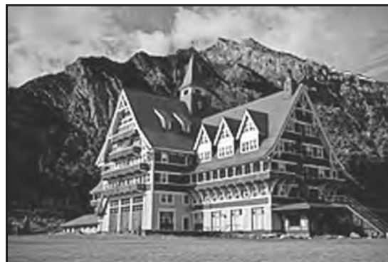
The Prince of Wales Hotel, Waterton Lakes National Park, Alberta, Canada, designed by Toltz, King, and Day and listed on the Canadian Register of Historic Places.
