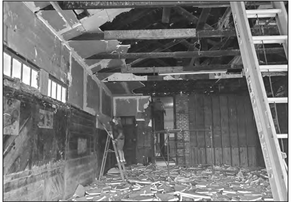
The entire inside of The Goodhue Depot needed to be torn apart and cleaned out. Most of the flooring was too damaged to save but the rest of the woodwork, the chimneys and doors were salvaged.
