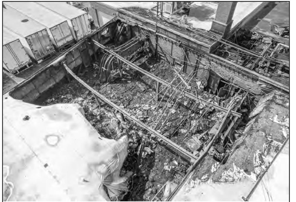
An overhead shot of the most severely damaged portion of the Hastings Creamery. The roof collapsed in this area as it was one of the hottest spots in the fire. This is where a good portion of the production was done at the plant. For reference, the photo through the side door is through the closed door on the upper portion of this image.
