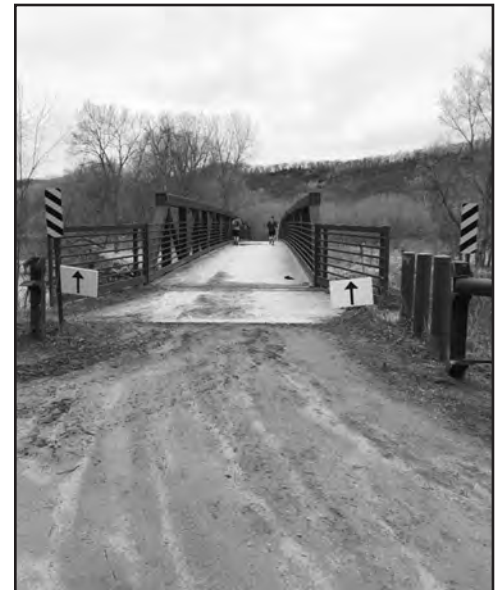
The bridge over the Zumbro
