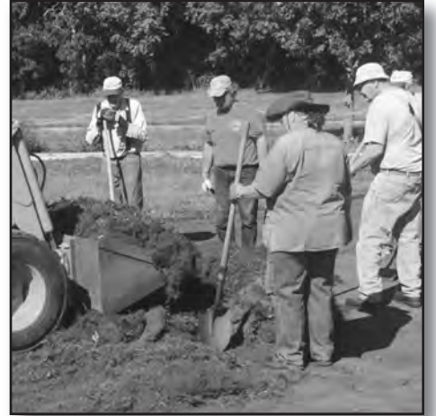
Rough Grading for Engine House
