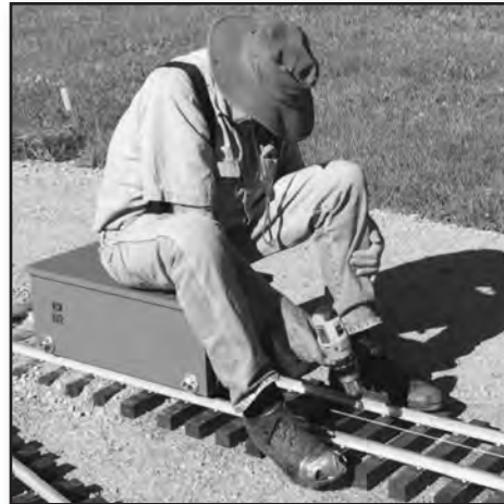
Final Tightening of Track Screws
