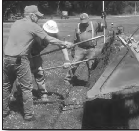
Placing Gravel for Roadbed
