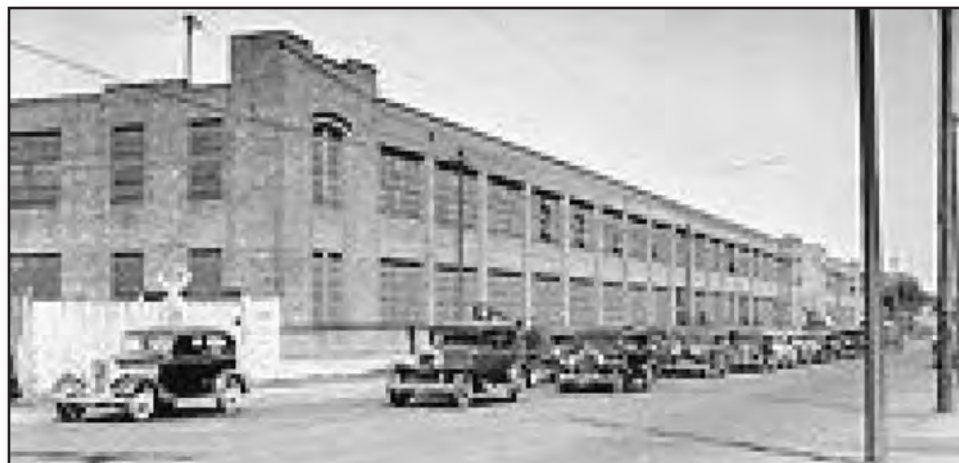
Minneapolis Moline, Lake Street and Minnehaha Avenue, Minneapolis, Minnesota Built 1902, Razed 1973
