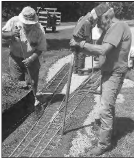
Placing Ballast
