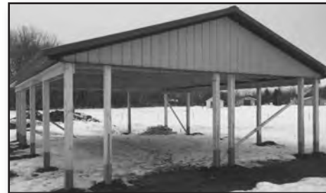
Framing for the Engine House
