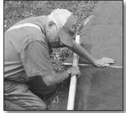
Final Level of Roadbed
