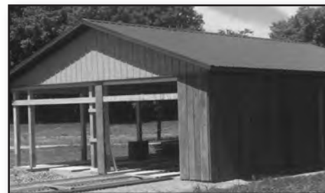
Partial Siding on the Engine House
