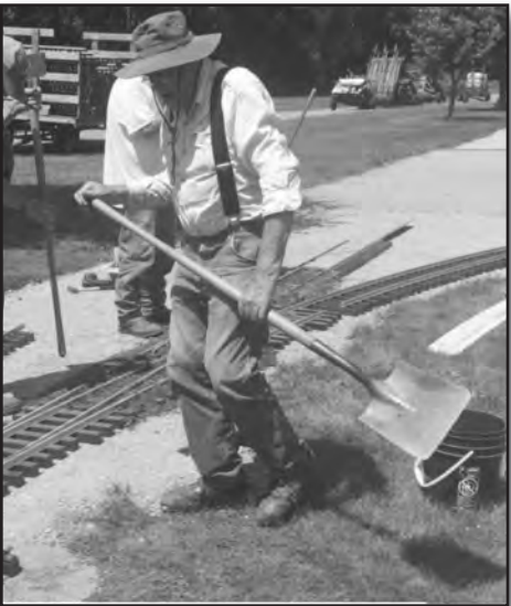
Setting the Track Sections
