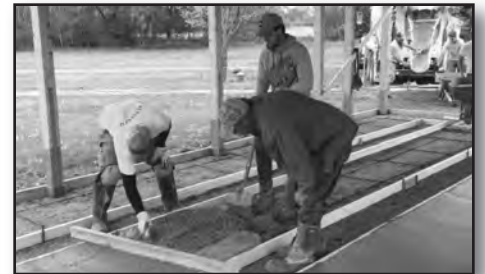
Pouring the Engine House Floor
