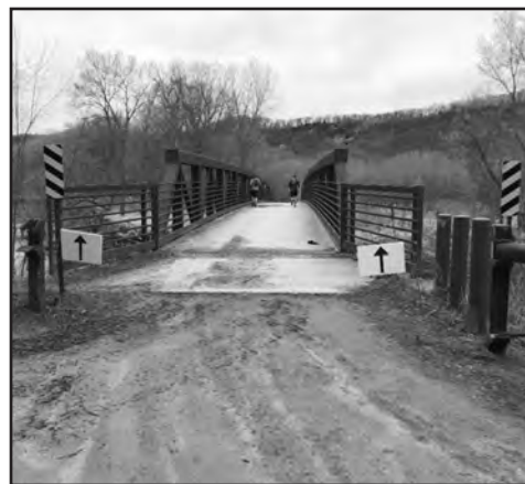
The bridge over the Zumbro
