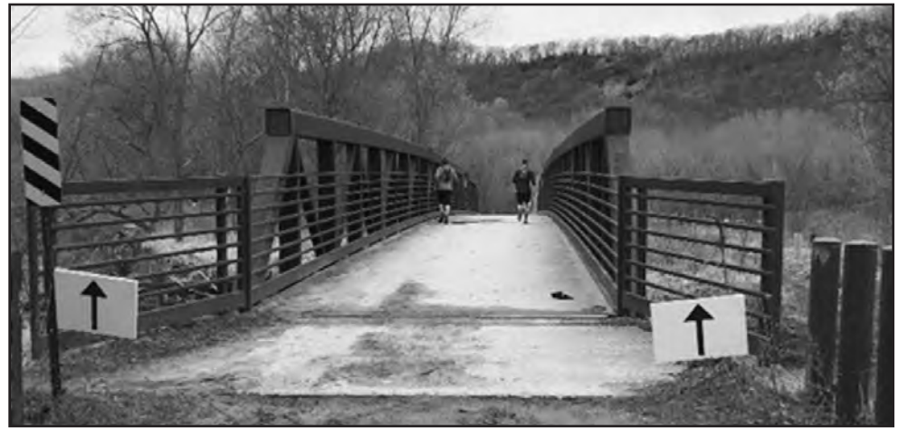
The bridge over the Zumbro
