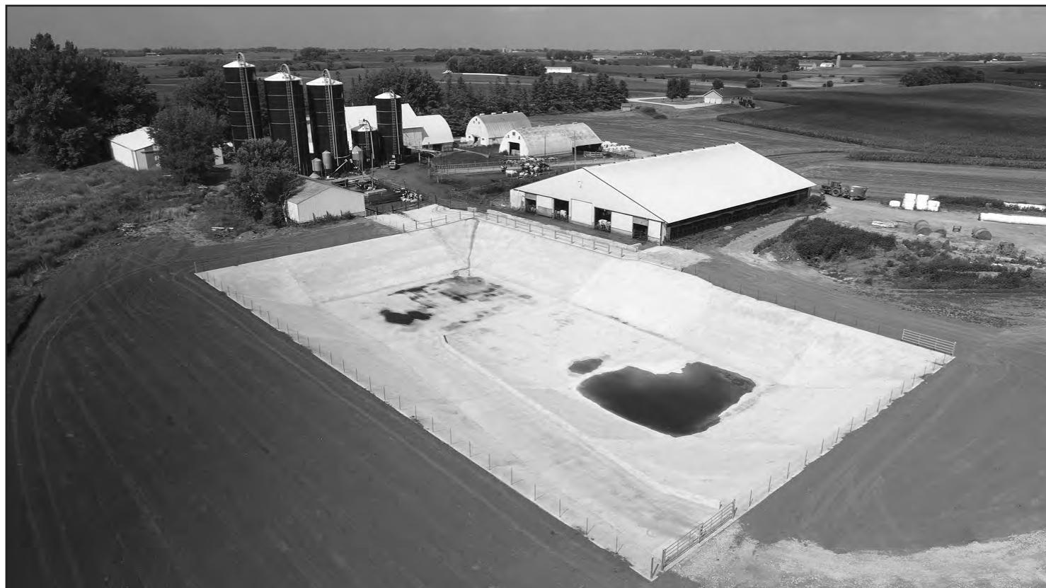
Watershed-Based Implementation Funding supported the feedlot upgrade on Tony Scheffler's Minneola Township dairy farm. The new manure pit has the capacity to hold 14 months of manure, which means Scheffler can apply that nutrient when conditions are right and the plants need it most. Photo Credit: Goodhue SWCD
