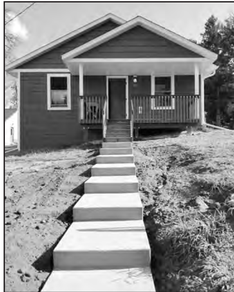
The Habitat for Humanity home on Park Avenue was built mainly by the Goodhue High School construction class.
