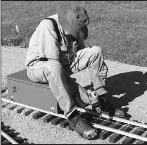
Final Tightening of Track Screws
