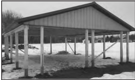
Framing for the Engine House
