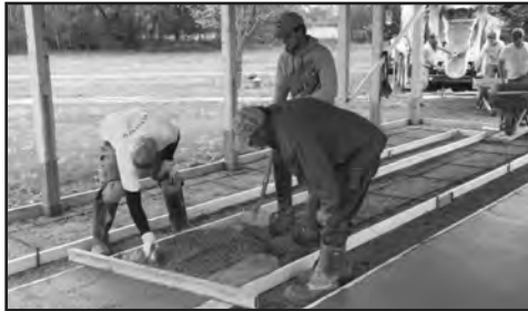
Pouring the Engine House Floor
