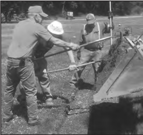
Placing Gravel for Roadbed
