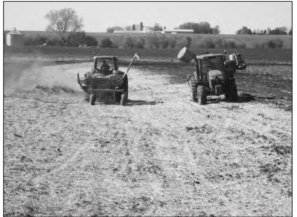
A newly constructed grassed waterway is seeded and mulched in Rice County.
