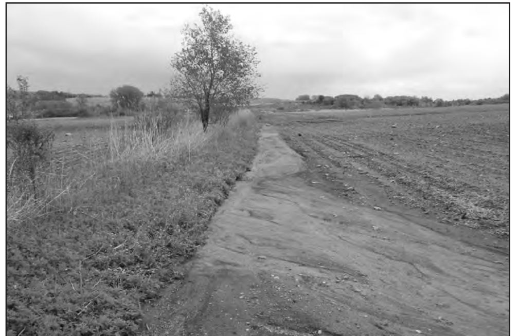
Volunteer trees and excess sediment collect by an unmaintained sediment basin in Rice County.
