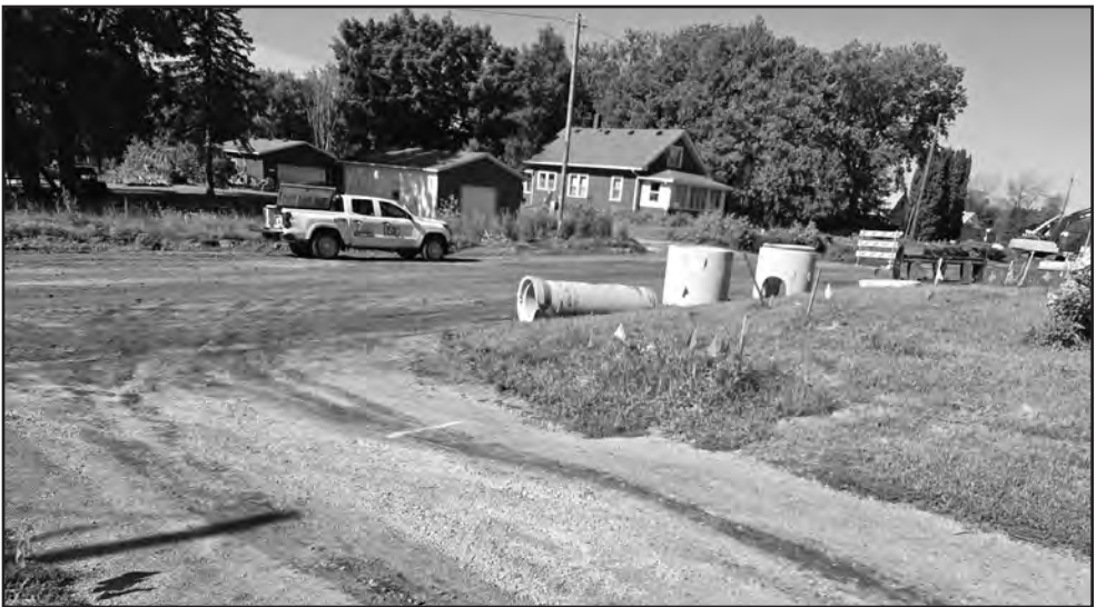
Lots of sizes went in to help pull water off Cty 86, along with storm drain collection ponds dug south of 86 also.
