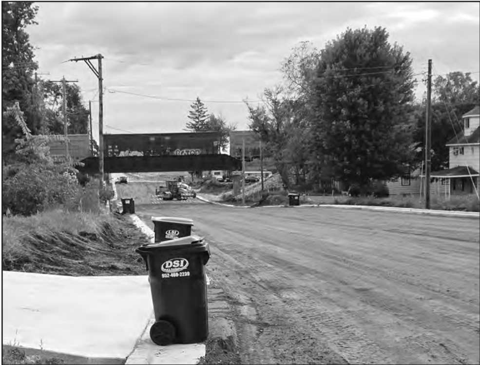
Castle Rock County Road 86 July 9 week of storm drain work.
