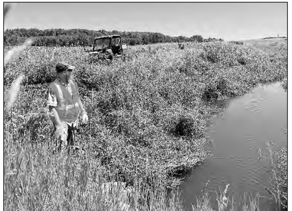
Ditch Manager Jarett Spitzack inspects a county drainage ditch in July 2024. Viewers have been hired to review public county ditches to equitable assessment of benefits.
