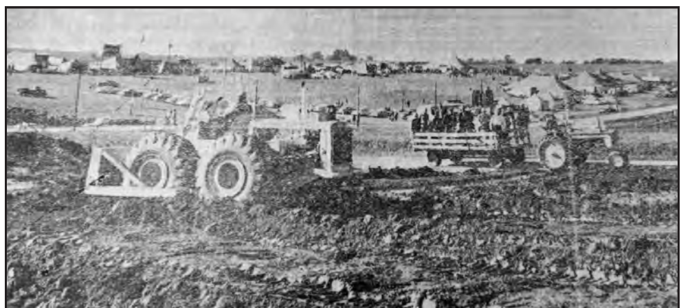
Here a bunch of spectators watch with interest the bulldozing of a new driveway on the Donald Dare farm. Background shot gives an excellent view of the headquarters area on the Peter Perrotti farm. photo courtesy of Rochester Post Bulletin
