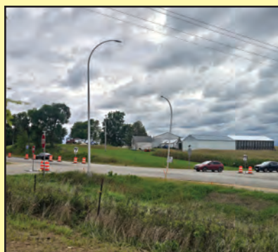
MN DOT installed new signage on Highway 56 and County Road 9 east of Dennison on Monday September 21st, 2026 converting the intersection to a four-way stop.
