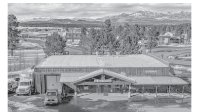
19 Navajo Trail Drive & The Buck Stops Here 6,800 sq. ft. building and business at busy intersection. Includes Koch Grand Prize smoker ($35,000 value), Cook Shack smoker, meat cutting equipment, meat grinder, band saw, meat rail system, scales, refrigerated display cases, meat tenderizer, meat slicer, tables, slaughter truck, freezer, cooler equipment. Seller will consider training and owner financing. All offers will be considered! Co-listed with Unger Realty
