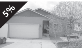
5% Upgraded Pagosa Lakes Home 134 Arrowhead Drive
