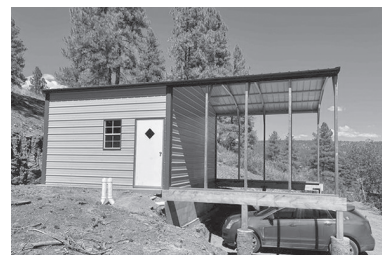
141 Hollow Drive 1.1 acres, no HOA, electric near, new engineered septic installed MLS 791781 • $79,900
