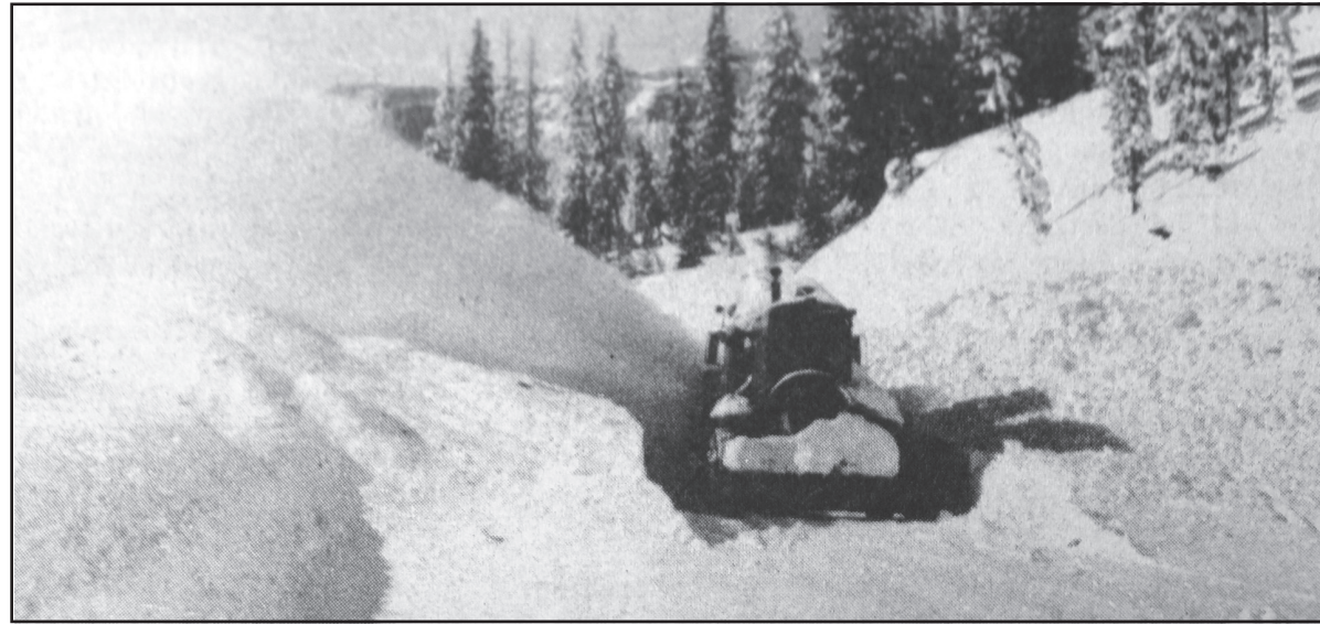
From the Dec. 29, 1983, Pagosa Springs SUN. BLOWING IT AWAY — Highway crews on Wolf Creek Pass needed four hours to clear a lane through Tuesday afternoon's avalanche. Wednesday morning this auger was widening the lane to make travel easier for motorists.
