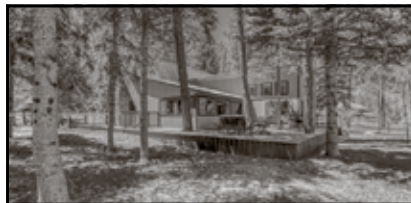
A Frame on the Rio Blanco River 344 Carrico Street
