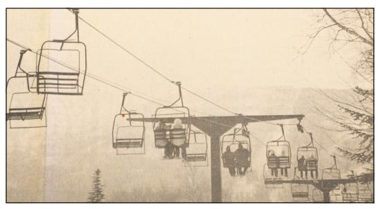
From the Sept. 5, 1974, Pagosa Springs SUN. READY SOON — A new, 1,000 skier-per-hour lift is being installed at the Wolf Creek Ski Area. This double chair lift is a first for Wolf Creek. It will replace a surface type lift installed in 1955. The base terminal of the lift is just a few feet from the ski lodge and the upper terminal sets right at the Continental Divide. The view from the lift will be breathtaking and skiers will have serveal runs available form the unloading terminal of the lift.
