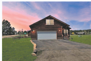
18 Snow Circle $369,000 Ranch style 4/2 home on fenced corner lot in Lake Hatcher area. MLS 769834
