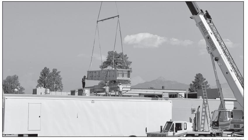
Photo courtesy Pagosa Springs Medical Center As part of its HVAC renovation project, crews hoisted a 7,000-pound HVAC unit onto the roof of Pagosa Springs Medical Center early last week.
