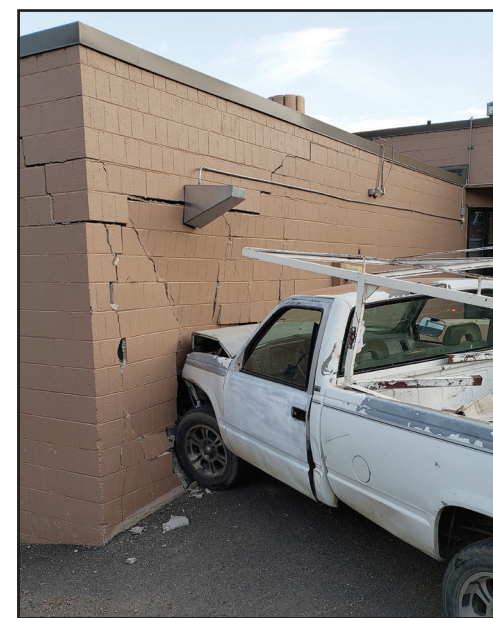
Photo courtesy Pagosa Fire Protection District
