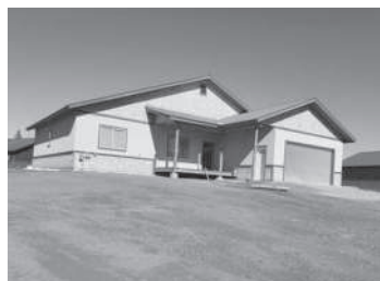
3B/2B under construction MLS 783608 - $649,000
