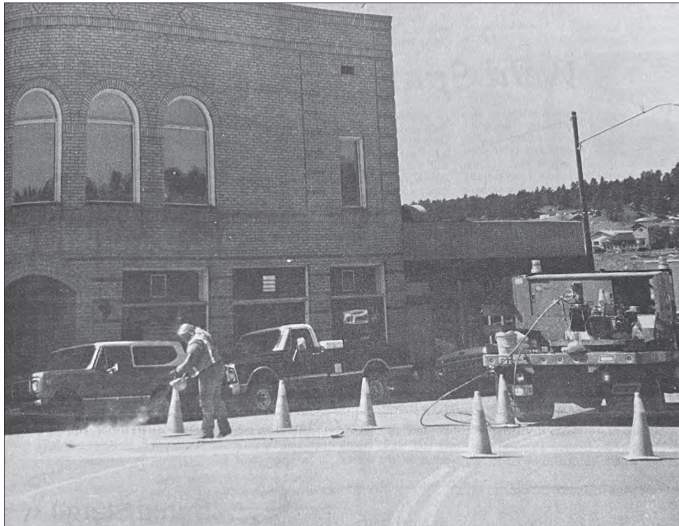
From the April 28, 1988, Pagosa SUN —SPRING SPRAYING — State Highway Department employee Melinda McCarty spent Tuesday afternoon applying fresh coats of paint to pedestrian crosswalks of Main Street. It is surprising how this type of service always gets done earlier in Pagosa Springs during election years.
