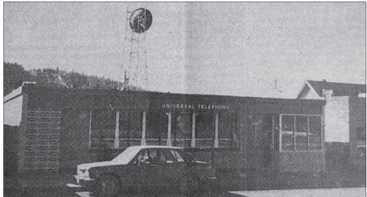
From the Aug. 24, 1978, Pagosa SUN — TELEPHONE OFFICE — This building houses Universal Telephone Co. in Pagosa Springs and is the central exchange office where new equipment has been installed to give telephone users in this area one party service. Direct distance dialing also became available this past week.
